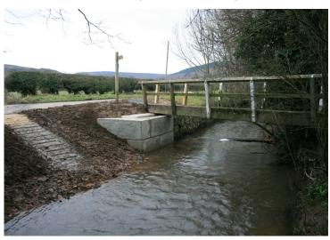
The footbridge over Potto Beck at the Gold Hill Loop road has now been repaired following flood damage last year and the footpath is now open. The new foundations have been prepared with a view to widening the footbridge when funding allows
